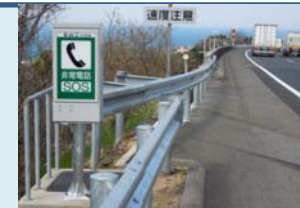
Emergency phone system
